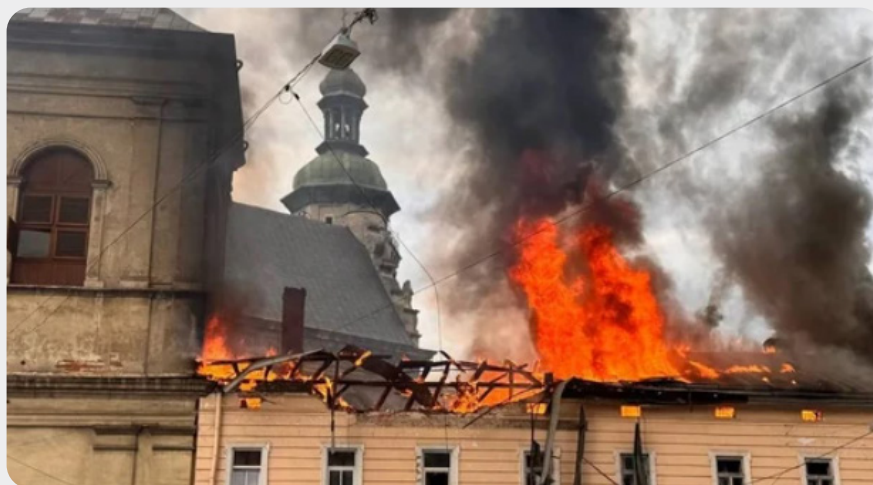
The Bernardine Monastery building in Lviv hit by a drone Source: Ukrainska Pravda .
