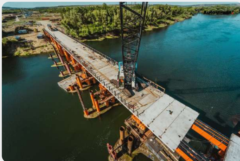
Construction of the new bridge in Vinnytsia oblast between Ukraine and Moldova The source is This is Vinnytsia, mate.
